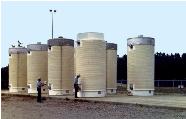
Dry cask storage
